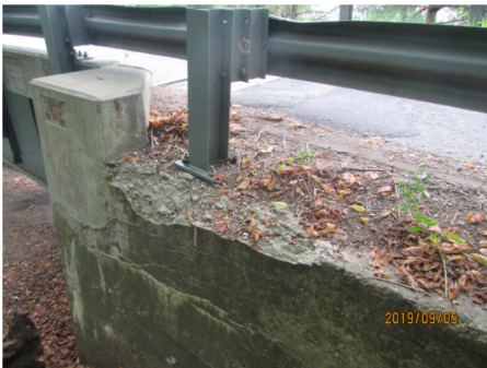
(NORTHWEST WINGWALL, ~ 8 L.F. REPAIR)
